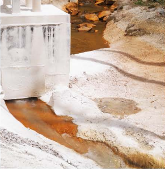
Acid mine runoff stains the streambed orange before it meets a lime doser at Maple Run, which sits in the Tygart Valley River watershed.
