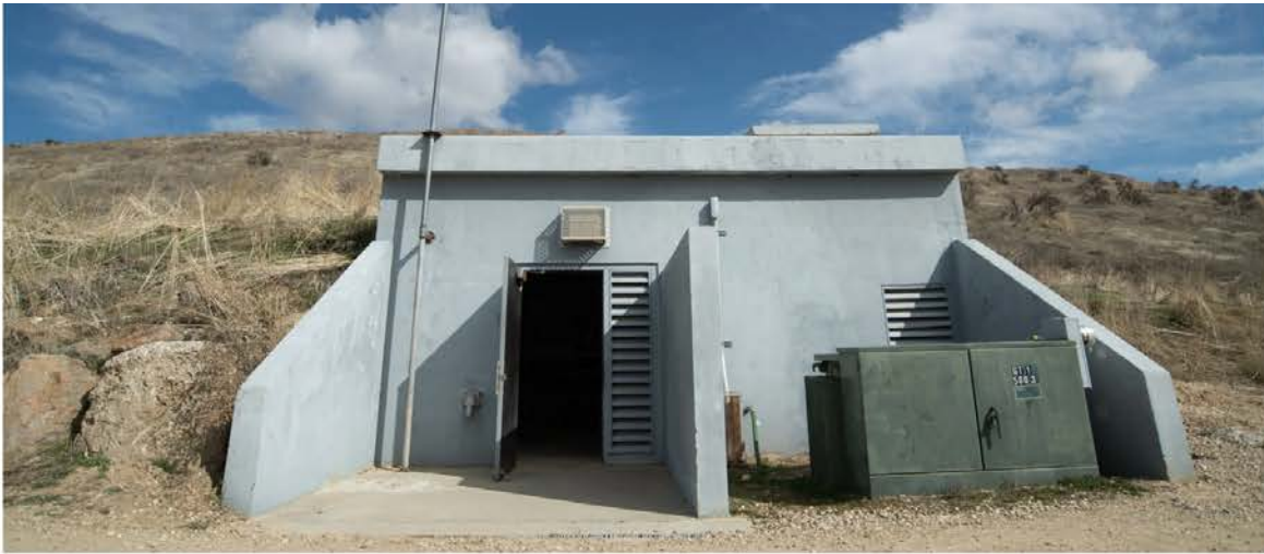
The main pump house serves as the control center for the three wells that make up Boise's geothermal system.
